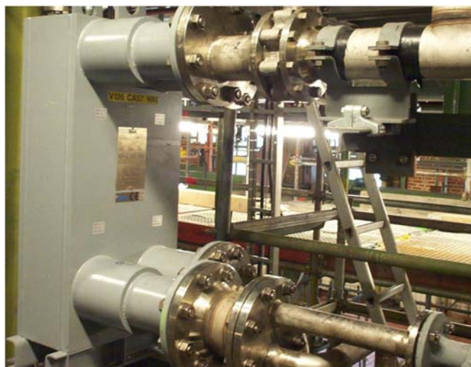
SIGMAWIG ST30 for steam condensation
